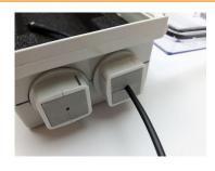
Push the gland in completely until it flush with the inlet.
